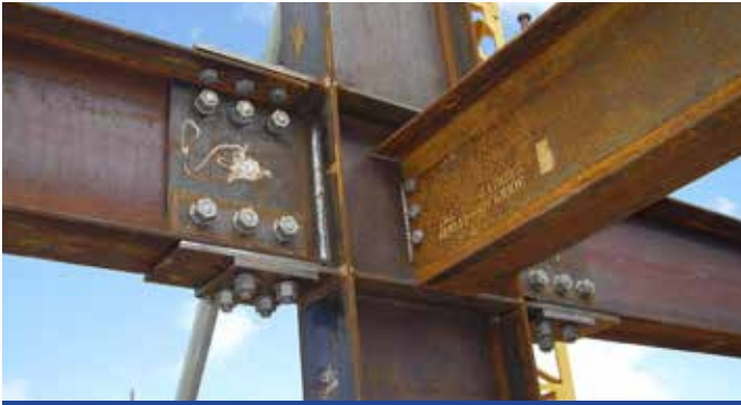
STEEL STRUCTURAL FITTING
