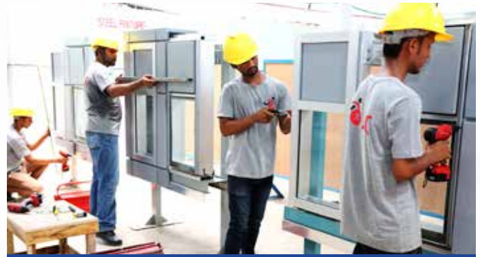
CURTAIN WALL INSTALLATION
